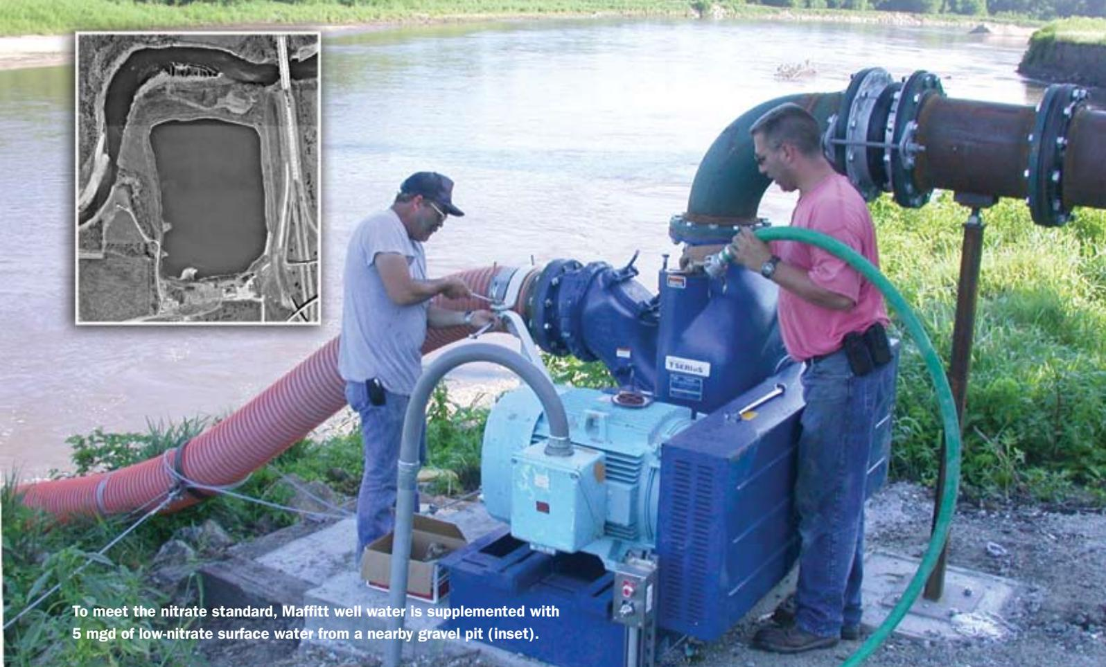
To meet the nitrate standard, Maffitt well water is supplemented with 5 mgd of low-nitrate surface water from a nearby gravel pit (inset).
